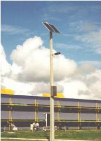
Figure 3-2. Pathway PV lighting system at Brevard Community College.
