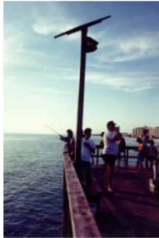
Figure 3-3. PV pier lighting (Panama City Beach, FL).
