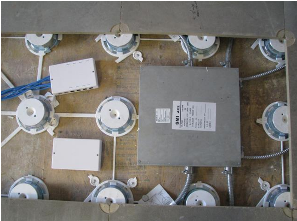
Low height access flooring with underfloor cabling
