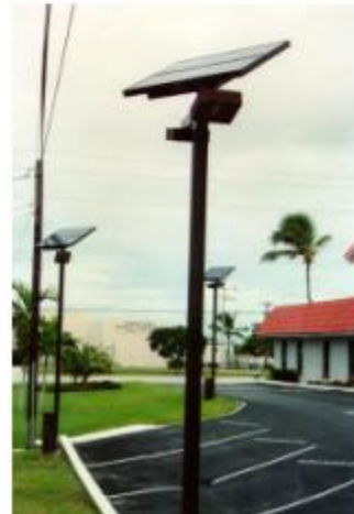
Figure 3-4. PV security lighting (Florida Keys).
