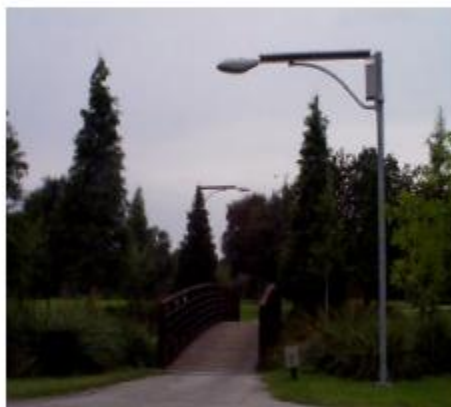
Figure 3-5. PV park lighting (Lakeland, FL).
