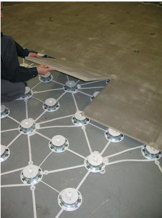
Underfloor Cabling Systems
